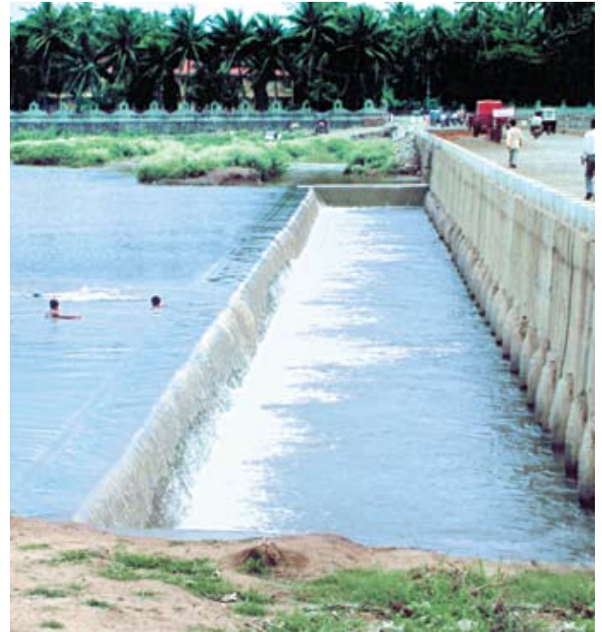
Check dam at river Malan
