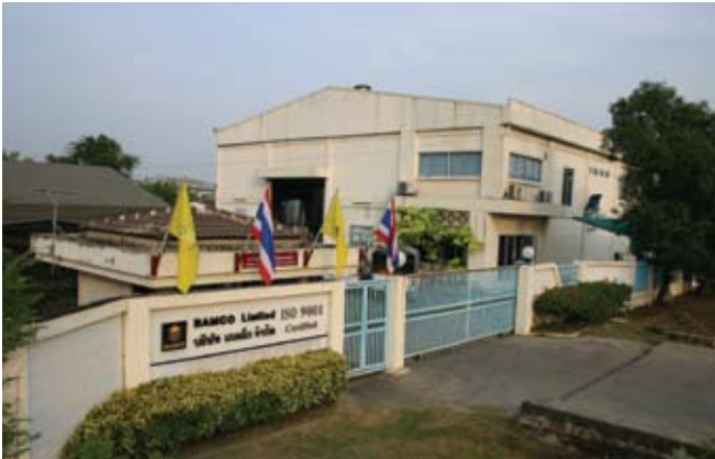
Pidilite Bamco manufacturing plant
