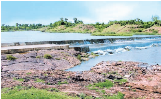
Check-Dam on River 'Malan' village Sangania
