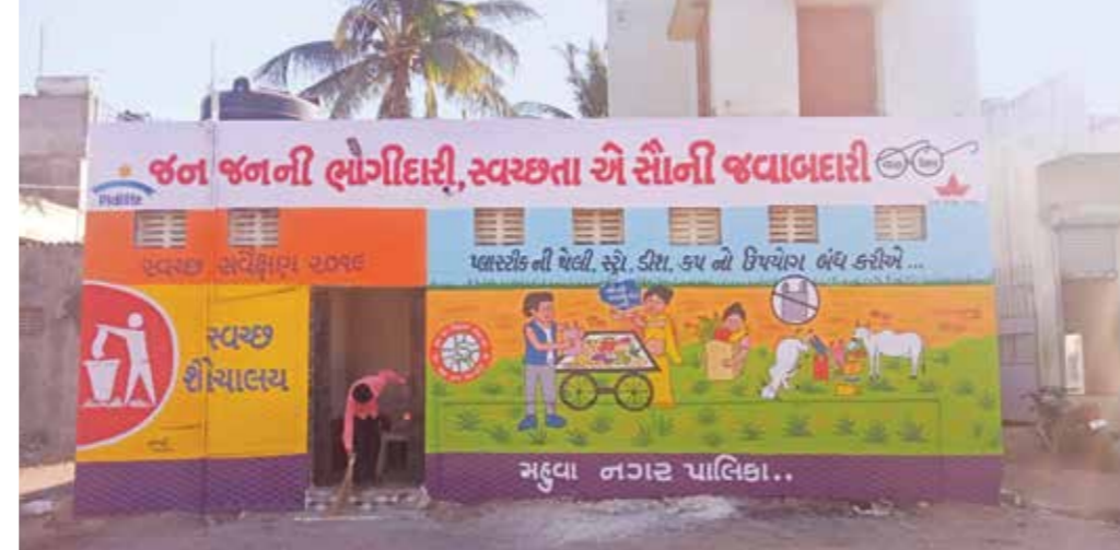
RENOVATION OF COMMUNITY TOILETS IN MAHUVA
