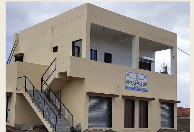
New SHG units being constructed
